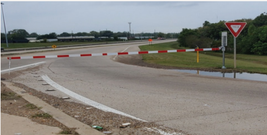
Figure 1. DOTD Contraflow Ramp Closure Gate
