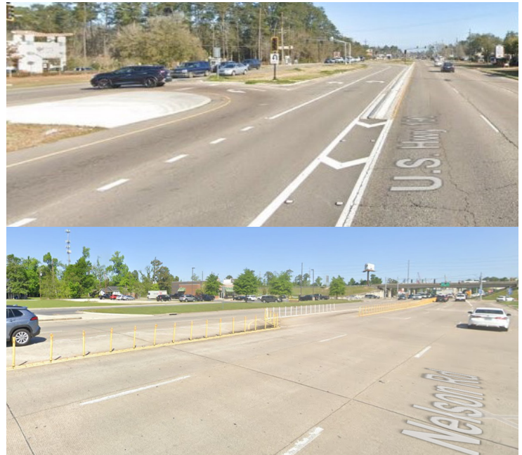
Access management treatments evaluated for economic impact in this project included J-turns (pictured at top) and raised curb channelization (pictured at bottom), among several others.
