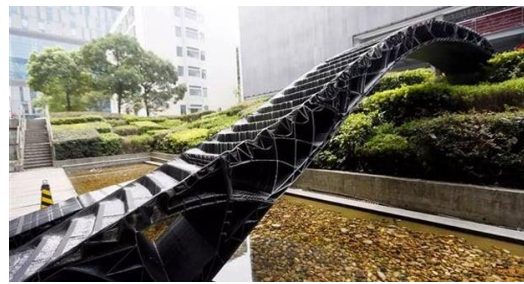
(b) Thermoplastic 3D printed bridge with Kuka robotic arm (Source: University of Shanghai, China)
