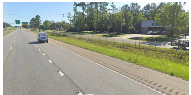
Figure 2. Access control fencing on US 90 [2].
