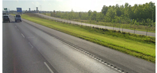
Figure 1. Access control fencing on I-10 [1].
