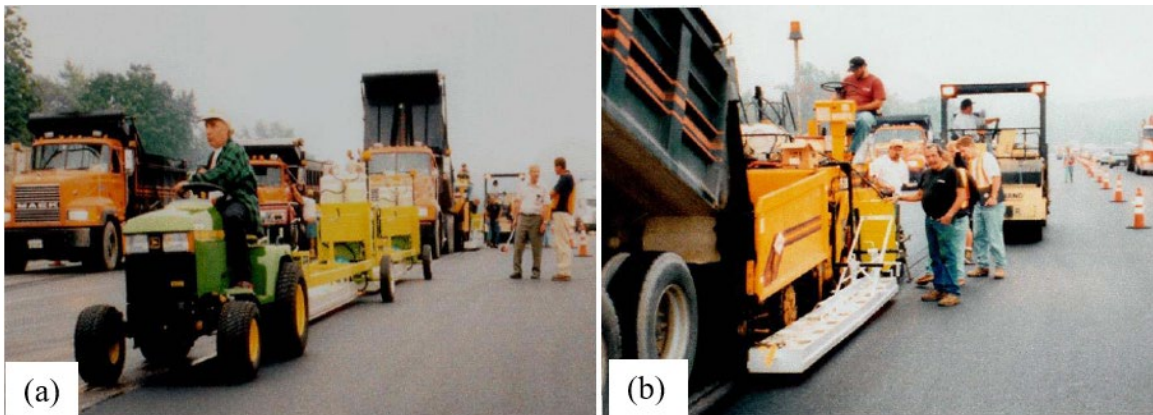
Figure 7. (a) Tractor-towed preheater and (b) paver-mounted heater (30)
