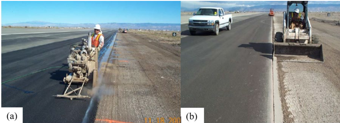
Figure 8. (a) Joint cutting and (b) removal procedure [33]
