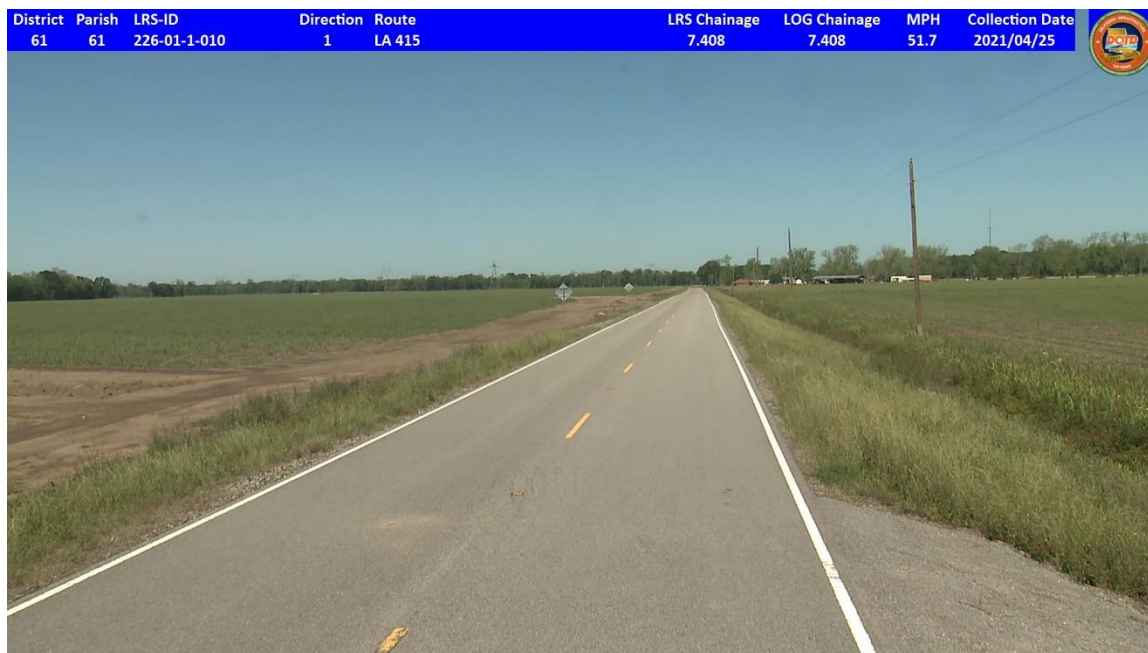
Figure 20. Right-of-way image for CS226-01
