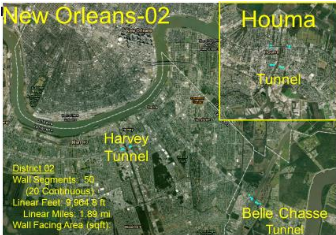
Figure 17. DOTD District 02 retaining walls
