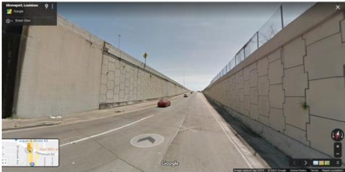
Figure 7. Mechanically Stabilized Earth (MSE) walls, Shreveport, LA
