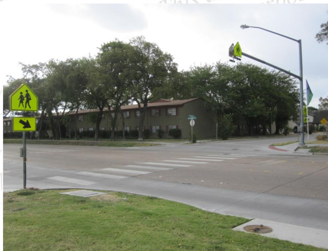
Figure 5. A crosswalk with RRFB and streetlight [83]
