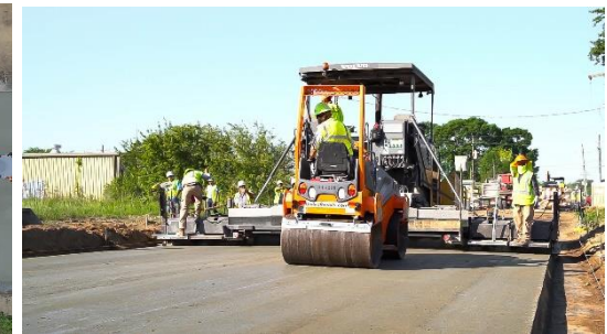
(f) Roller Compaction
