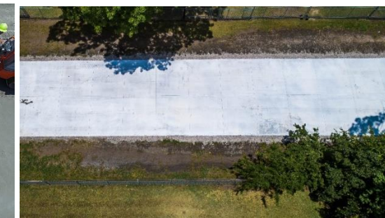
(h) Final surface after curing and saw-cut
