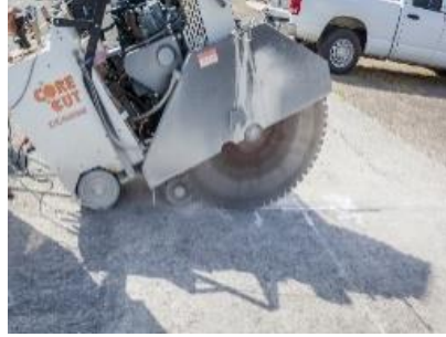
(a) Saw cutting
