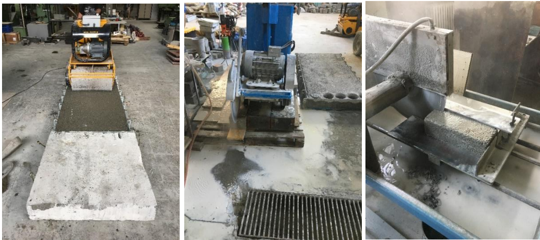
Figure 7. Preparation of RCC beam specimens.
