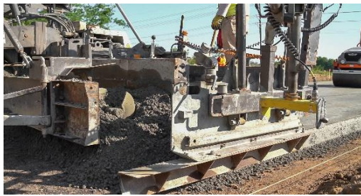
(c) Placement of RCC
