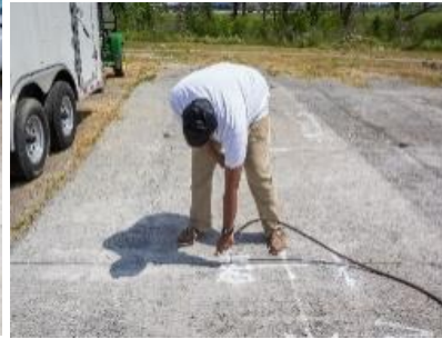
(b) Cleaning of saw cut
