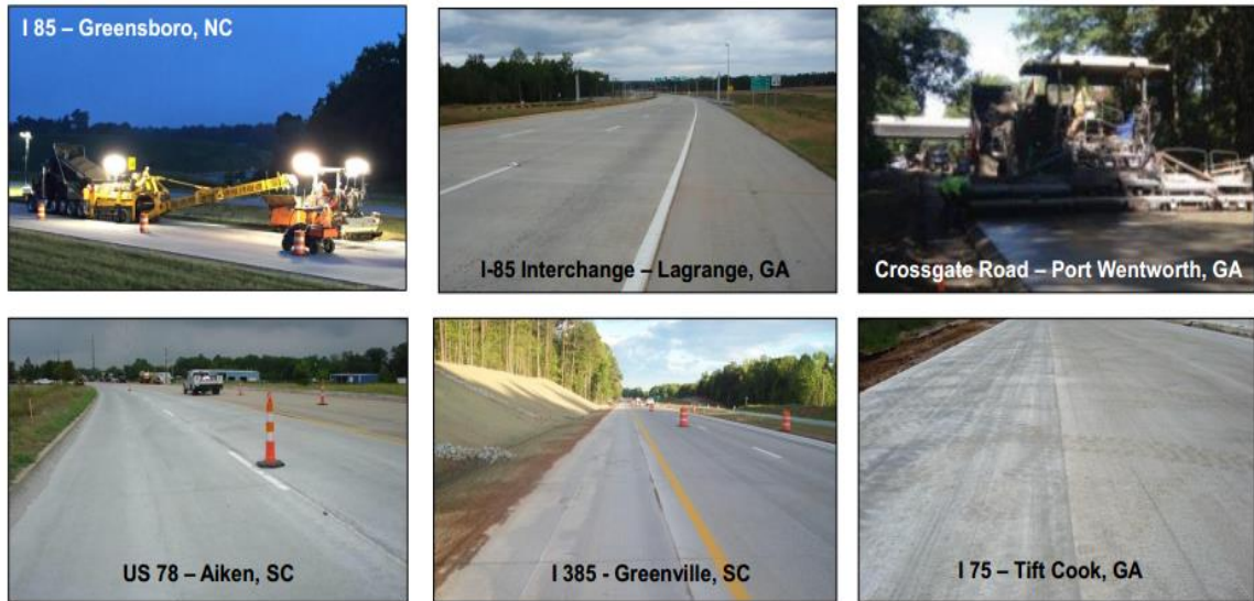
Figure 3. RCC application as shoulder and surface roads [31]
