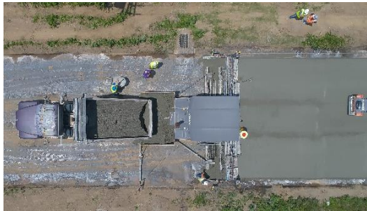
(e) Paving Operation
