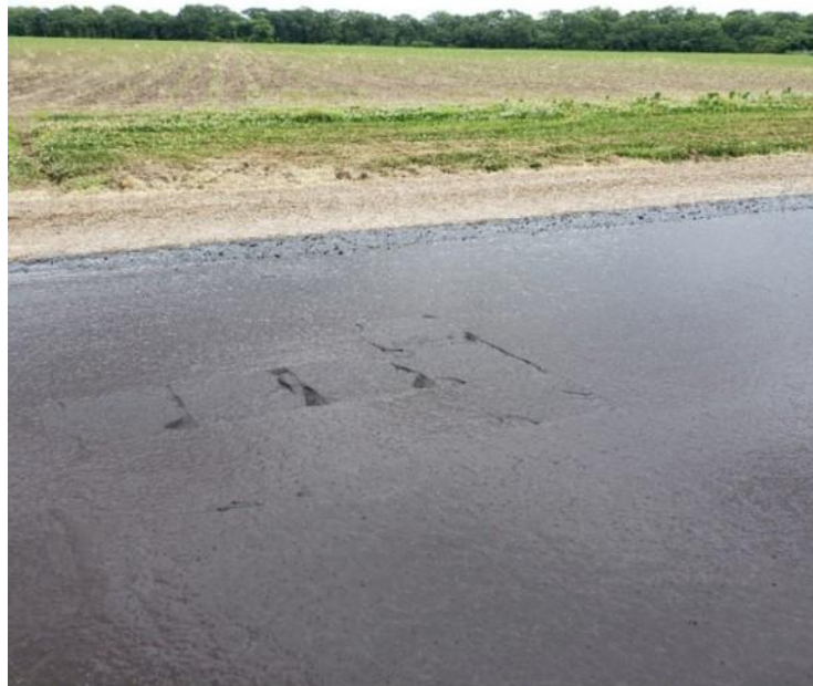
Figure 30. Geotextile pads after application of emulsion
