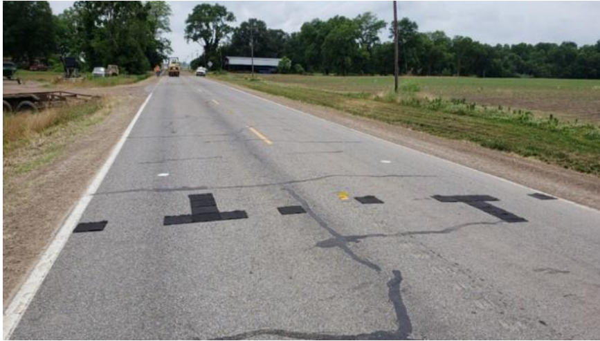
Figure 29. Geotextile pads placement on the test sections
