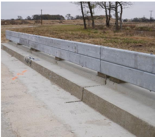
(c) Upstream of joint
