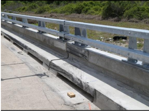
(a) Traffic face of bridge rail
