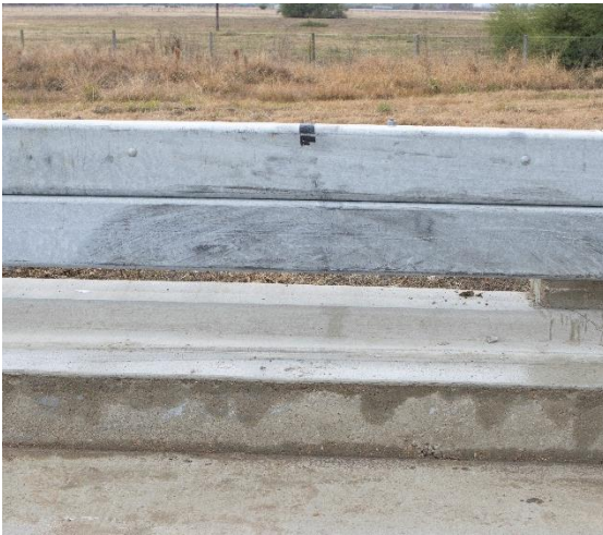
(c) Traffic side of posts at joint
