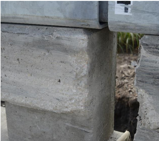
(c) Traffic side of posts at joint 4
