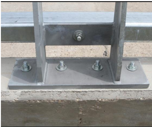
(e) Field side of post connection
