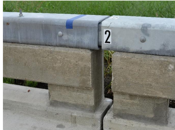
(b) Concrete parapet at joint 2
