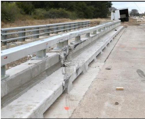
(a) Traffic face of bridge rail
