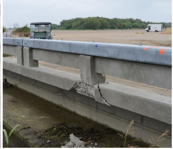
(b) Field side of middle post of section 2
