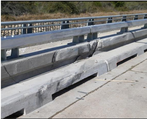
(a) Traffic face of bridge rail
