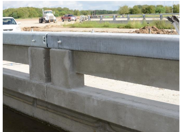
(b) Field side of joint 4
