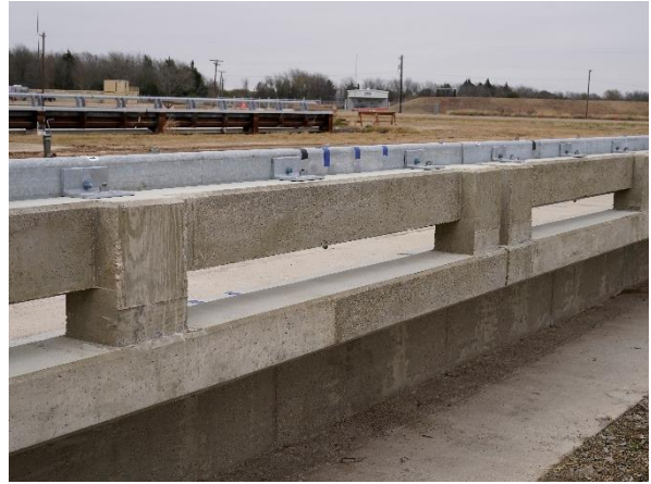
(b) Field side of bridge rail
