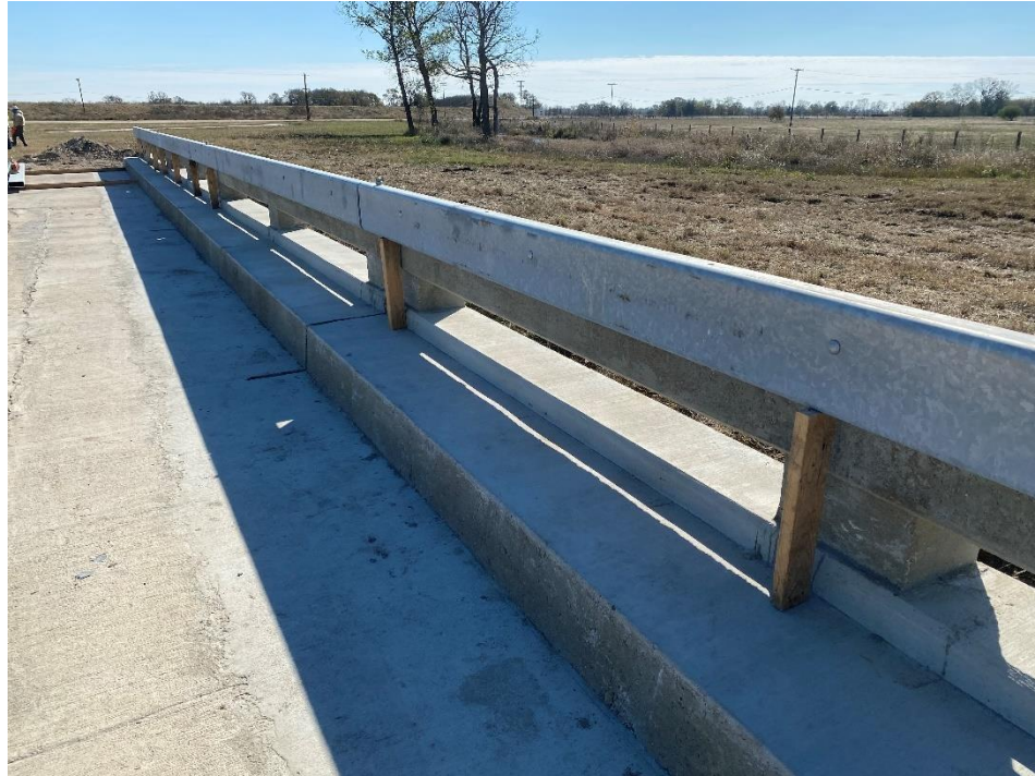
Figure 95. Installation of first/top rail element with temporary shoring support
