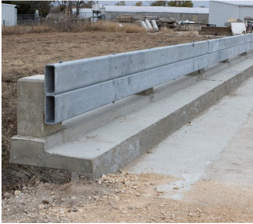
(a) Traffic face of bridge rail
