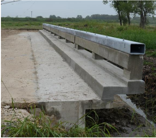
(a) Traffic face of bridge rail
