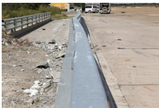
(b) Parallel with bridge rail
