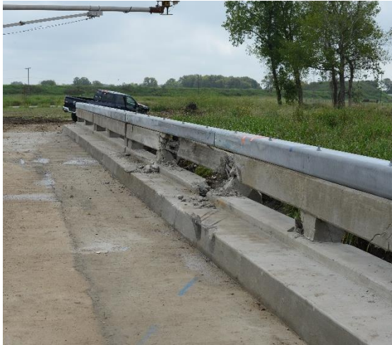
(a) Bridge rail/test vehicle after test
