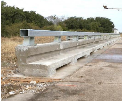
(a) Traffic face of bridge rail
