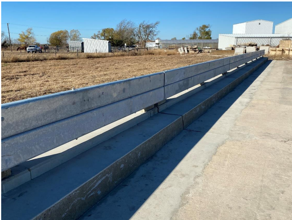
Figure 98. Front view completed retrofit rail installation
