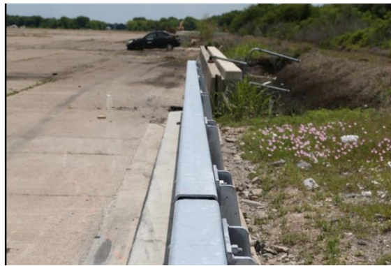
(b) Parallel with bridge rail
