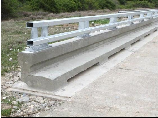
(a) Traffic face of bridge rail
