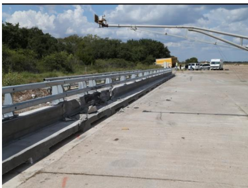
(a) Traffic side of bridge rail
