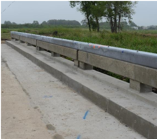
(c) Upstream of joint
