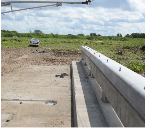
(a) Bridge rail/test vehicle after test
