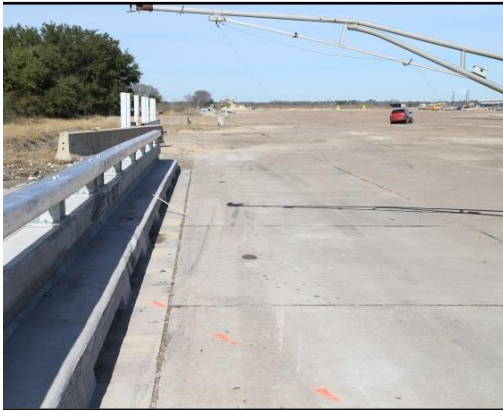
(a) Traffic side of bridge rail
