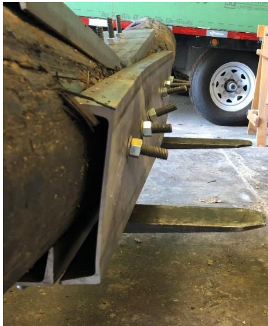
Figure 109. Yielding of bolts in C-channel splicing
