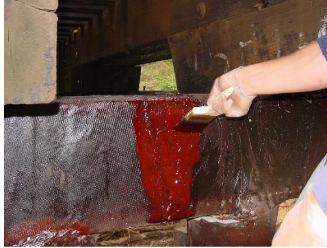
Figure 23. Sealing with phenolic
