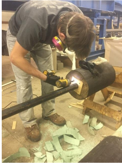
Figure 47. Setting timber for rehabilitation
