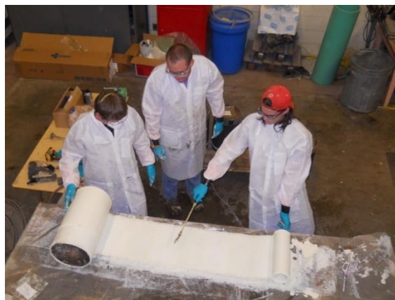
Figure 31. Spraying of Aquawrap for bond testing
