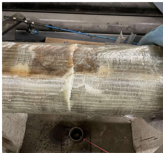
Figure A-3 – Compressive failure of fabric
