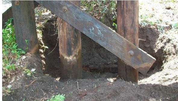
Figure 18. Pile excavation
