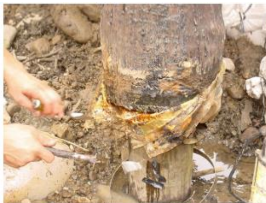
Figure 20. Removal of decay
