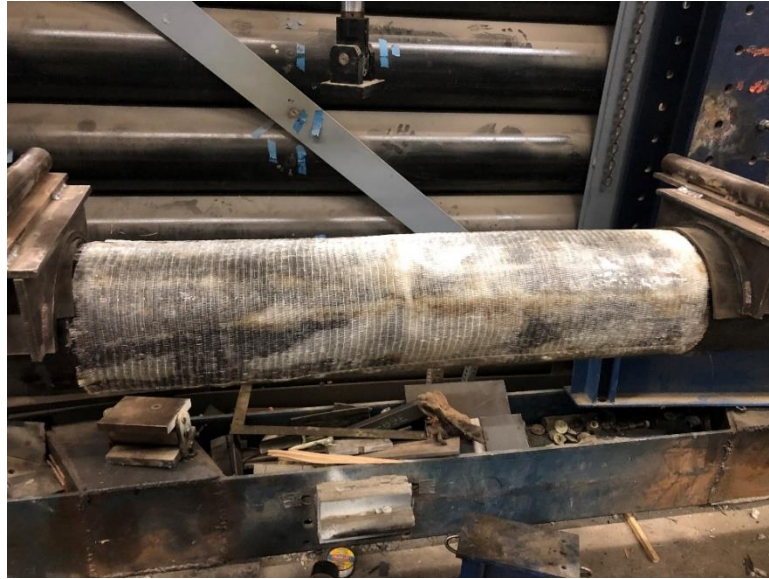
Figure 61. Completed fiber reinforced polymer splice
