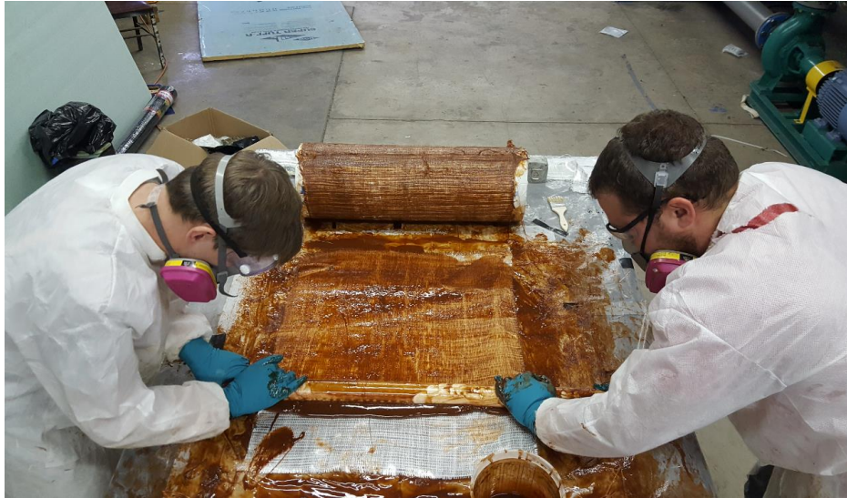
Figure 43. Saturating fabric and spreading resin
