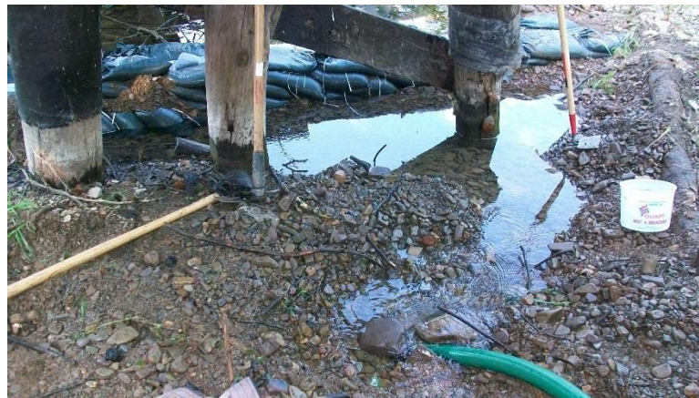
Figure 19. Removing excess water
