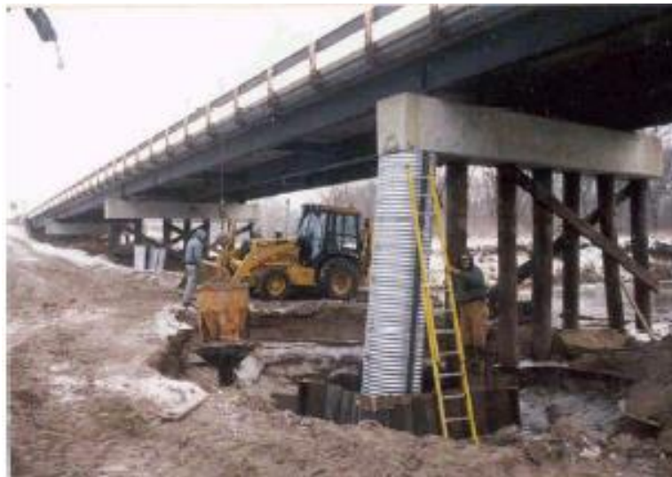
Figure 2. Concrete jacketing installation
