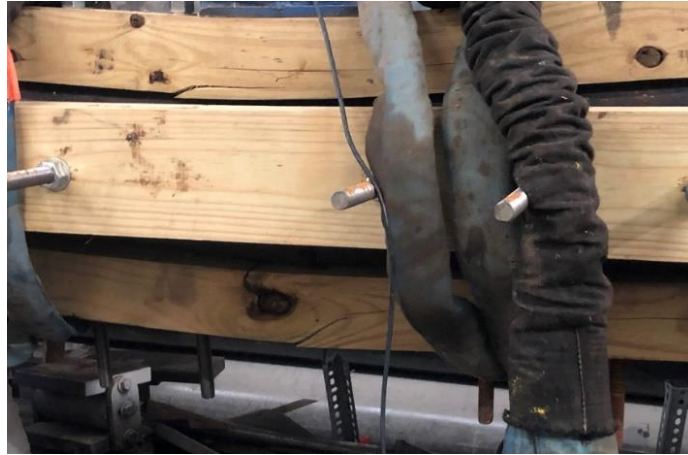
Figure 110. Cracking of top and bottom plates in wood splicing
