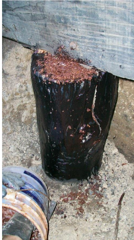
Figure 22. Primed and filled pile section
