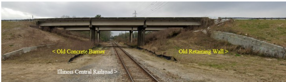
Figure 24. I-55 slope repair site prior to construction
