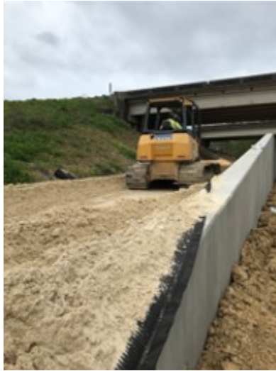
a. South retaining wall
