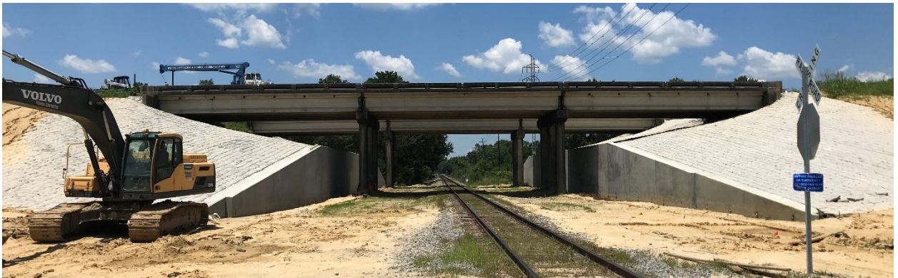
Figure 26. I-55 embankment wall completion
