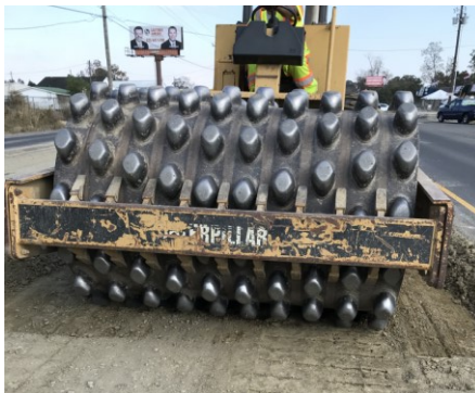
Figure 12. Pad foot roller for compaction
