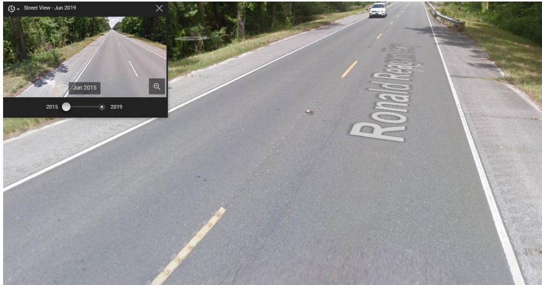
Figure 2. A Segment with both CLRS and SRS that has been Verified Using Google Street View
