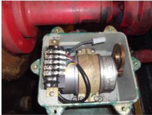
(a) Bridgeport selsyn opened for inspection
