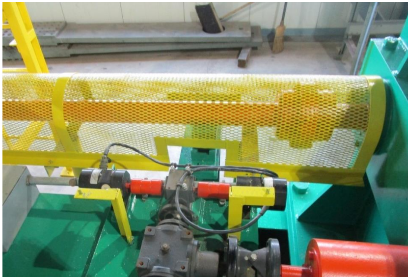
Figure 9. Skew control resolvers installed at Route 88 in Point Pleasant, NJ
