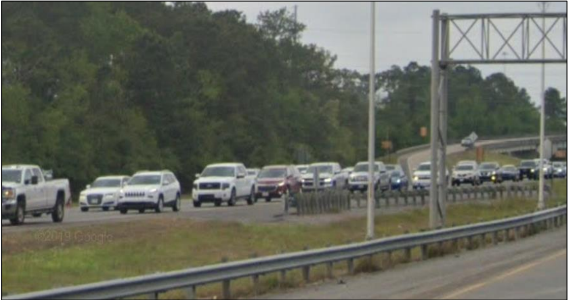
Figure 33. Queue back up due to work zone
