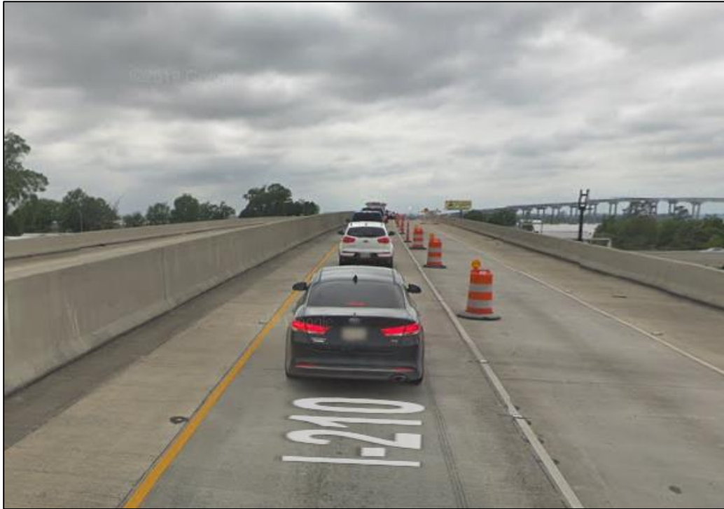
Figure 31. Right lane closure on I-210
