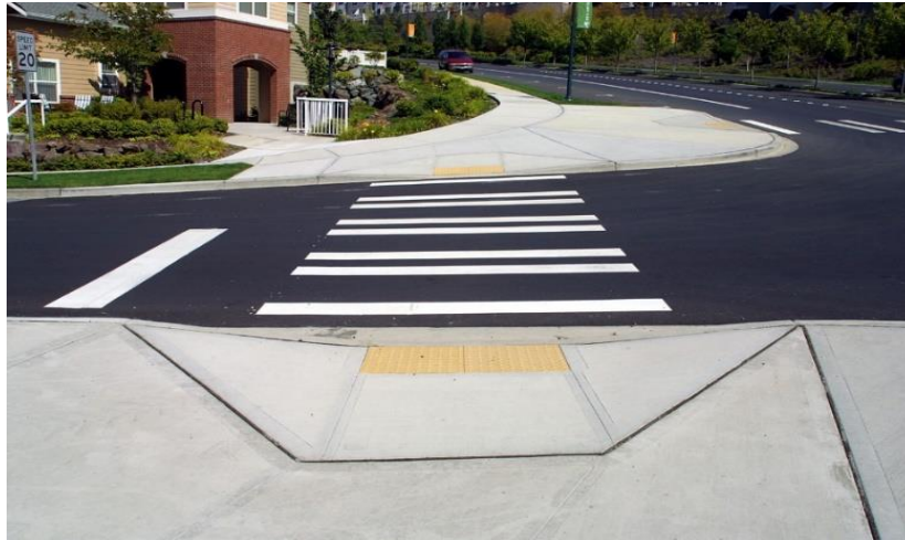
Figure B2. Pedestrian curb ramps
