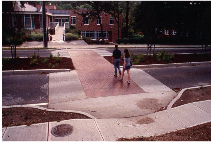
Figure B6. Raised pedestrian crosswalk
