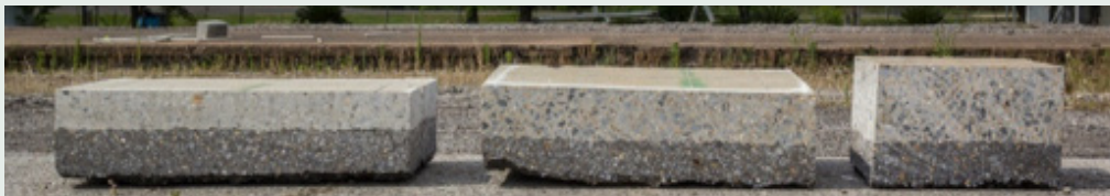
Figure 3 Forensic trenches of BCOA pavement sections
