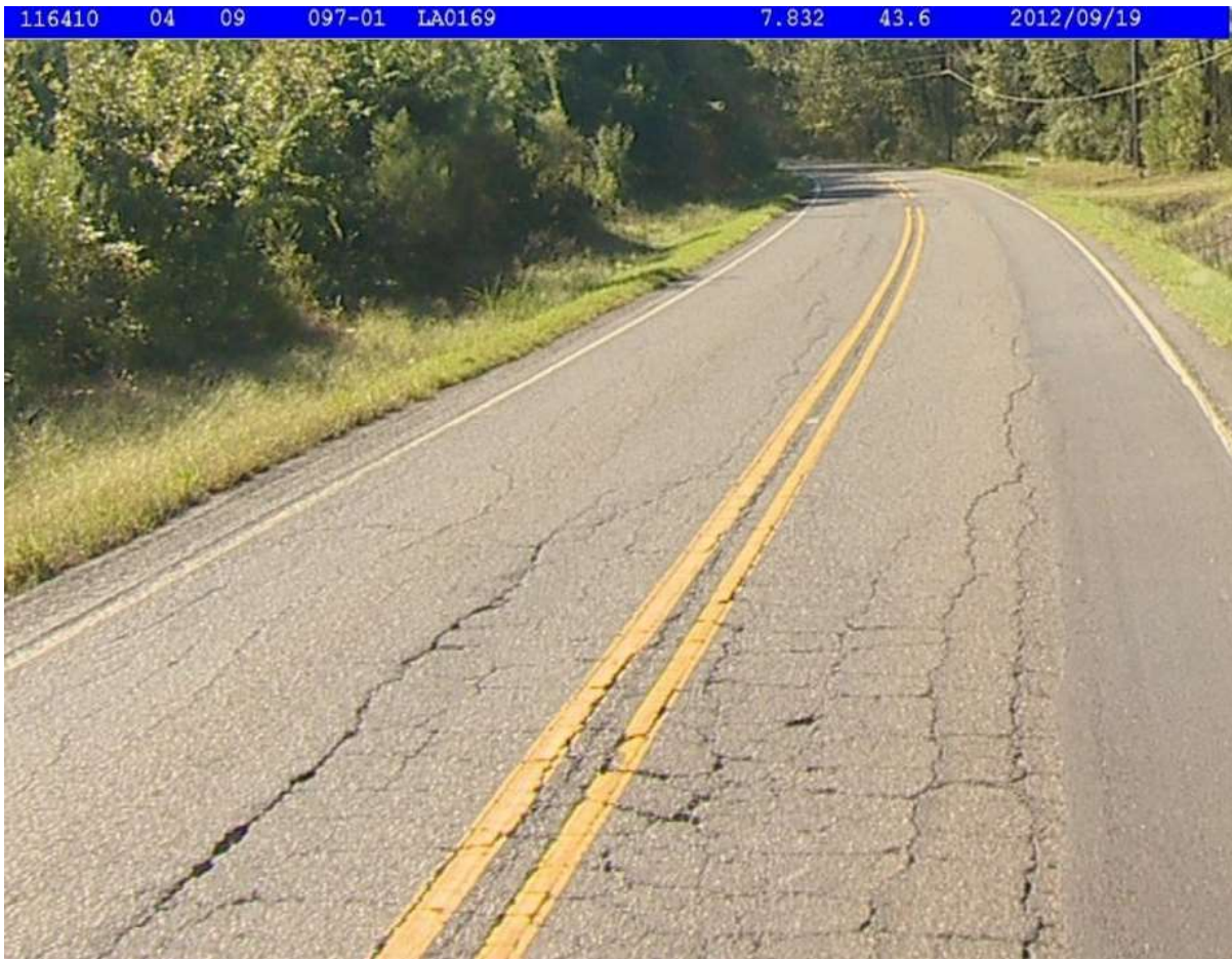
Figure 7 On-site view of LA169 in the area of Haynesville shale play
