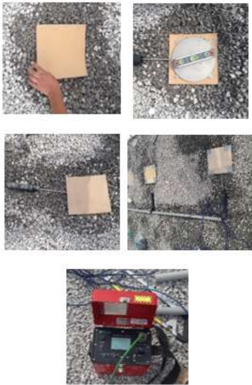
a) Installation of pressure cells
