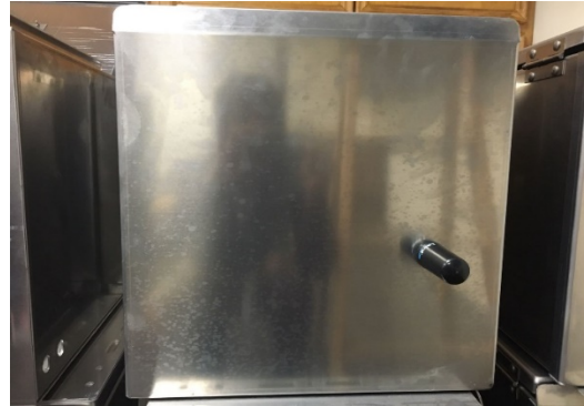
Figure 18 (a) Microhard Bullet-LTE cellular modem (b) antenna of cellular modem attached to cabinet
