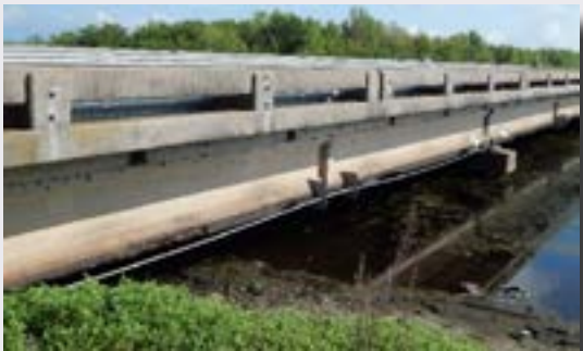
Figure 1 Distance view of the eastbound bridge
