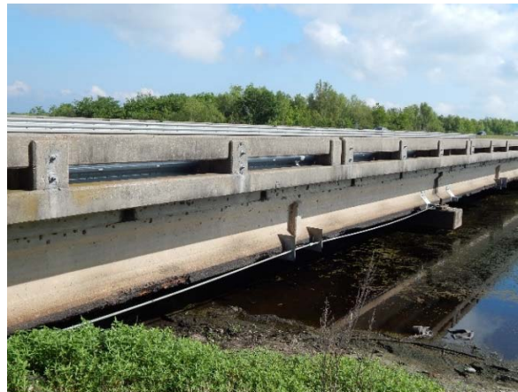
Figure 2 (a) Distance view of the eastbound bridge
