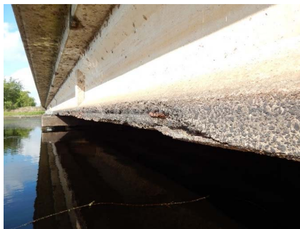
Figure 2 (b) Close view of the westbound bridge
