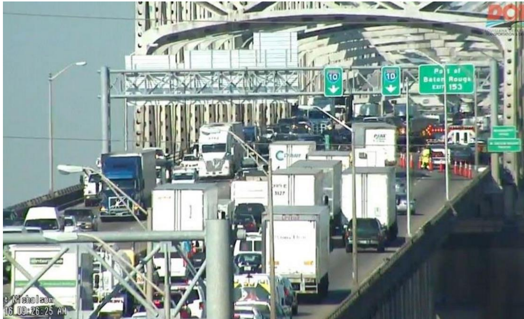
Figure 2. I-10 Mississippi River Bridge.
