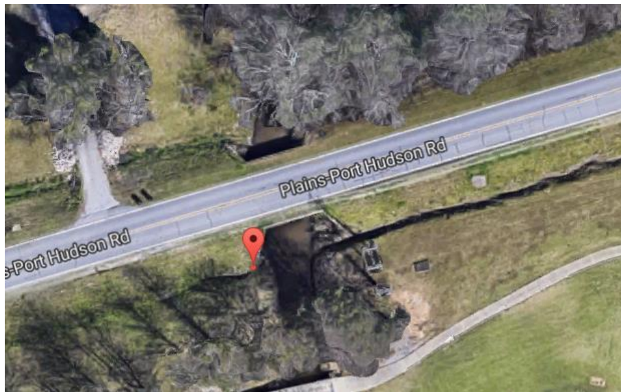
Figure A-2 Aerial view of Culvert #1 – Zachary, LA
