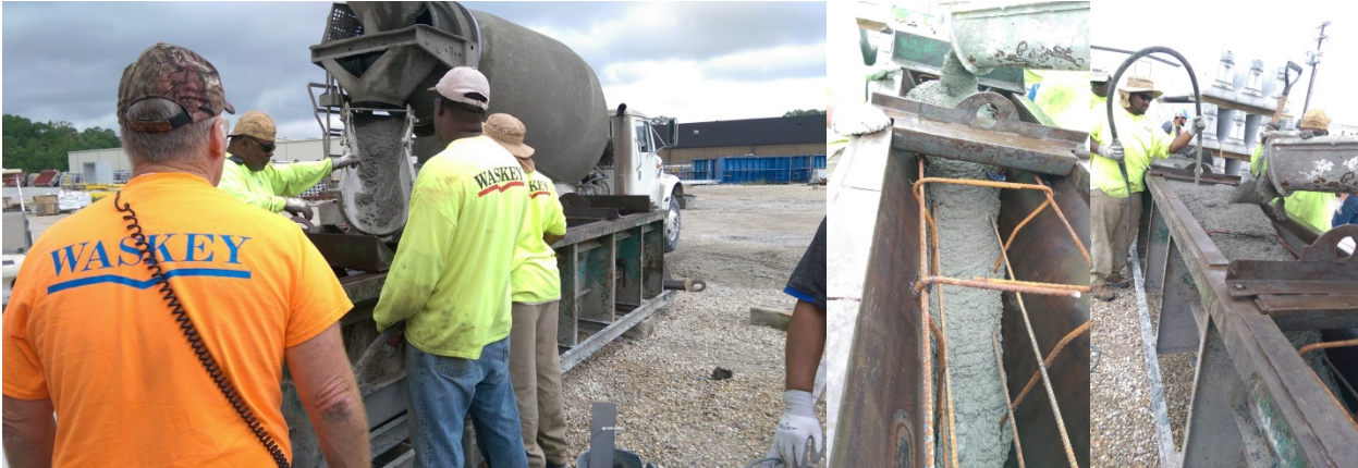
Figure 11: Pouring the barrier at the Waskey facility in Baton Rouge, LA
