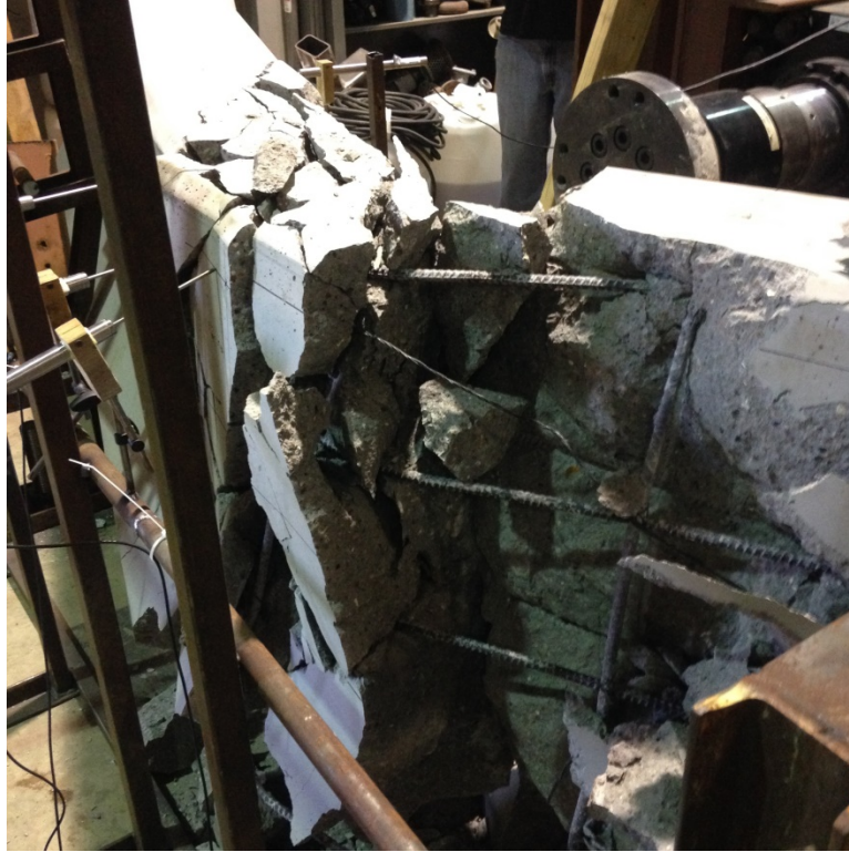
Figure 24: Tensile side of the barrier after complete crack and crush
