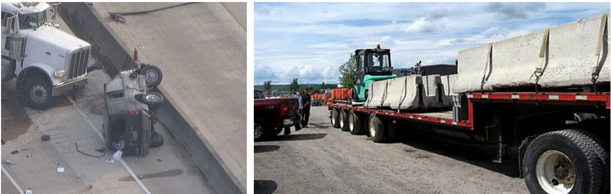
Figure 25: Barrier for traffic diversion and carrying of pre-cast barrier
