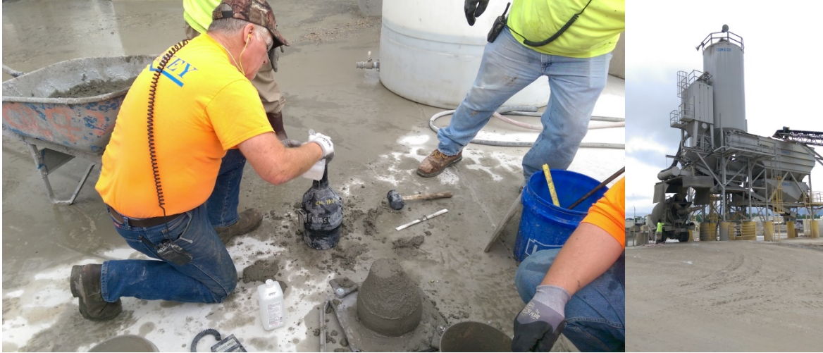
Figure 10: In-situ property testing & loading the concrete truck at the Waskey facility in Baton Rouge, LA
