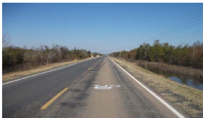
Figure 19 Coring test section Site 12 [14]
