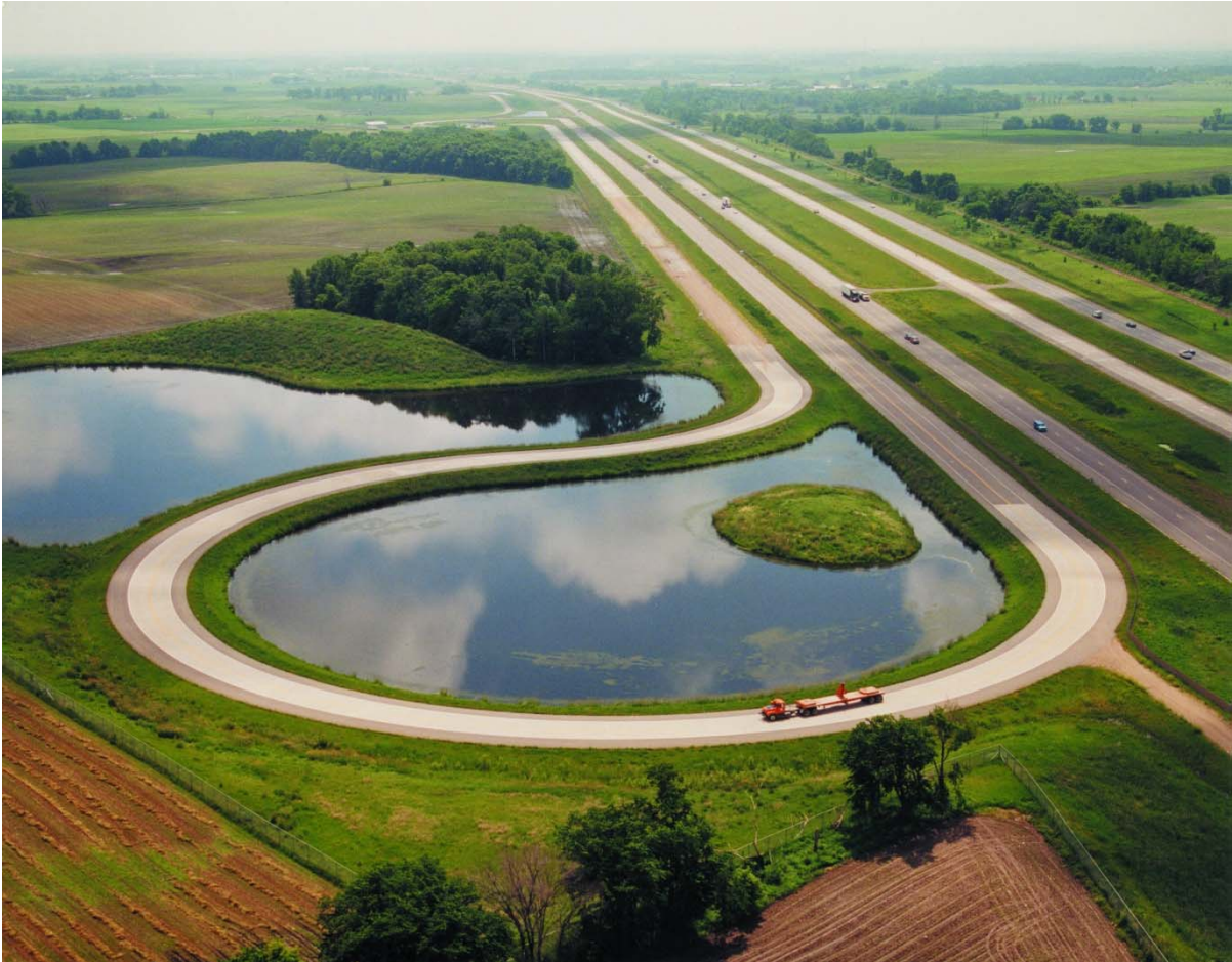
Figure 23 Overview of the MnROAD facility
