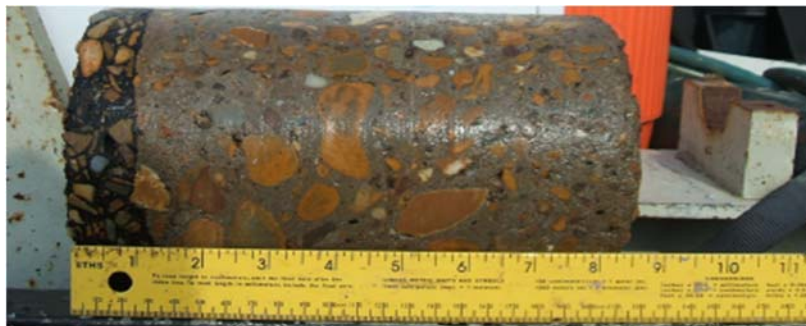
Figure 31 Example of core sample in good structural conditions (Section 182-01)
