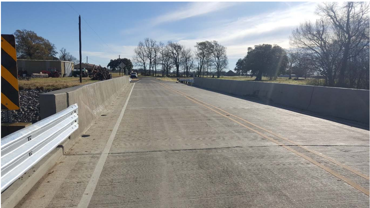
Figure 9 Completed West Congress Bridge looking east into Lafayette Parish
