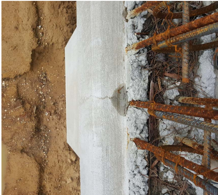
Figure 18 Picture of a crack over a column on the U.S. 80 bridge deck
