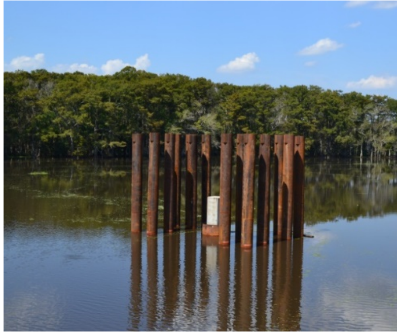
Figure 5 Load frame arrangement for TP-2 at Bayou Lacassine site
