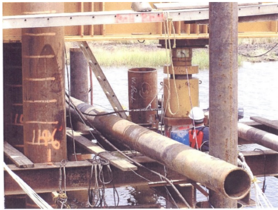
(a) Test site 2
