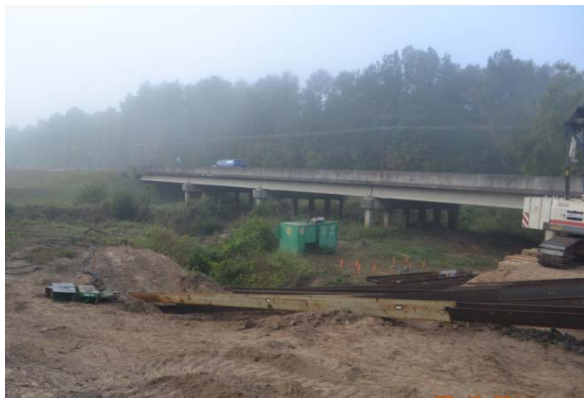
(a) Construction site
