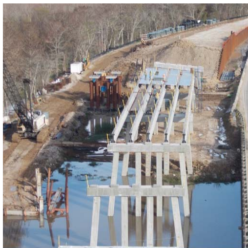
(a) Construction site
