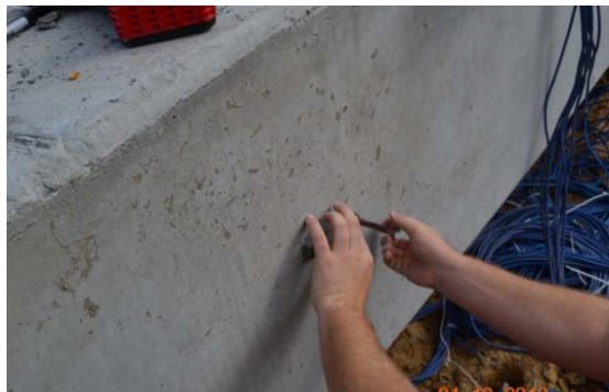
(e) Installation of accelerometer and strain transducer
