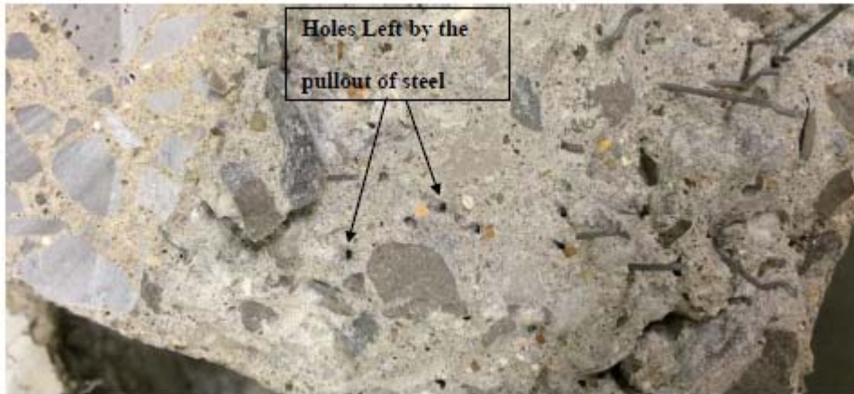
Figure 34 Example of hole left behind by steel fiber pulling out
