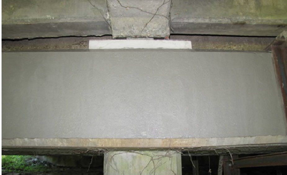
Figure 9 Initial coating with short discrete fiber reinforced composite
