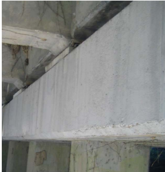
Figure 25 Close up of short fiber composite coating
