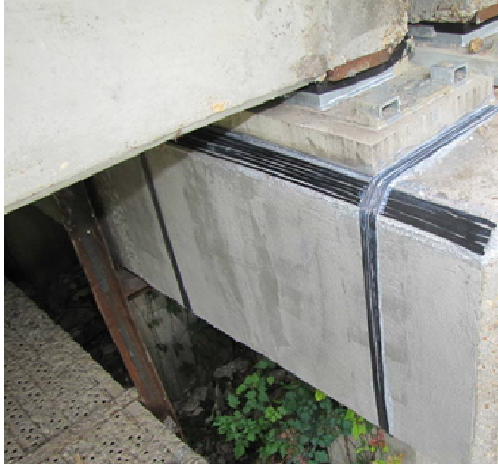
Figure 11 Details of the confining reinforcement
