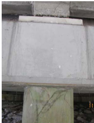
Figure 31 View of high modulus confinement composite: Continuous carbon tows can be seen on both sides of the bearing plate
