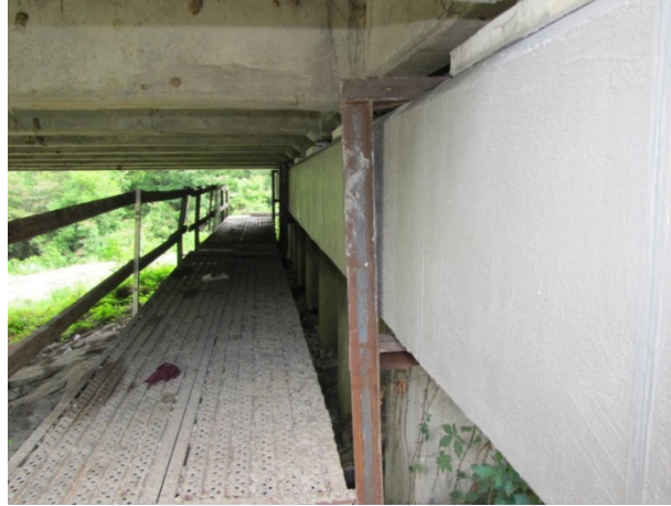
Figure 20 Appearance after the completion of second coat
