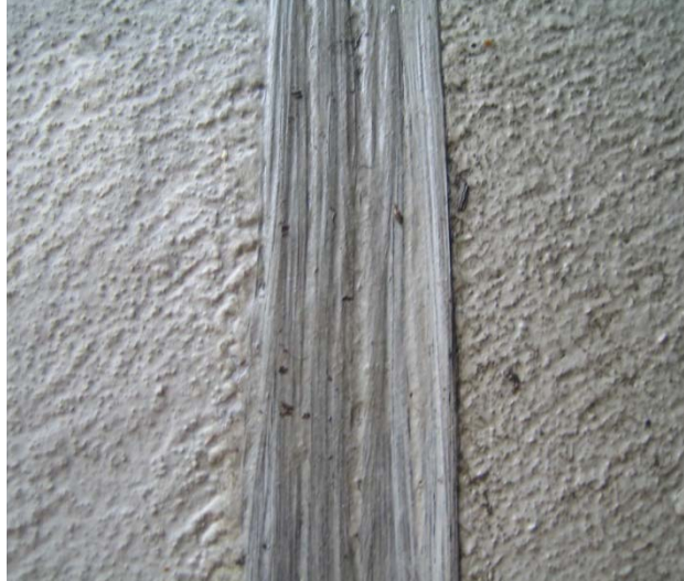
Figure 36 Close-up of carbon tows
