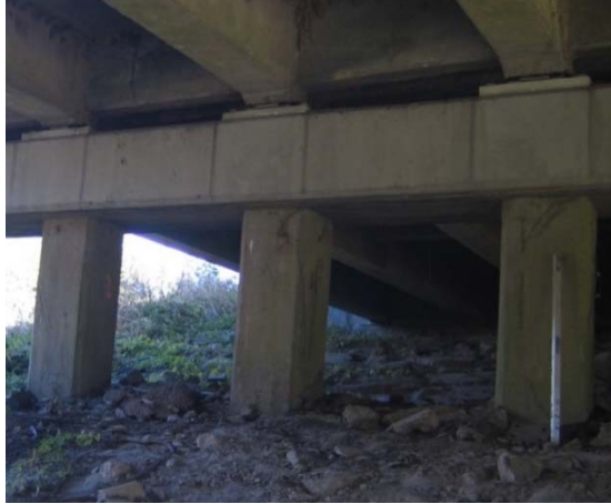
Figure 24 View of the overall structure
