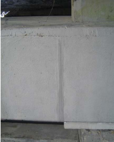
Figure 23 Close up of carbon tows
