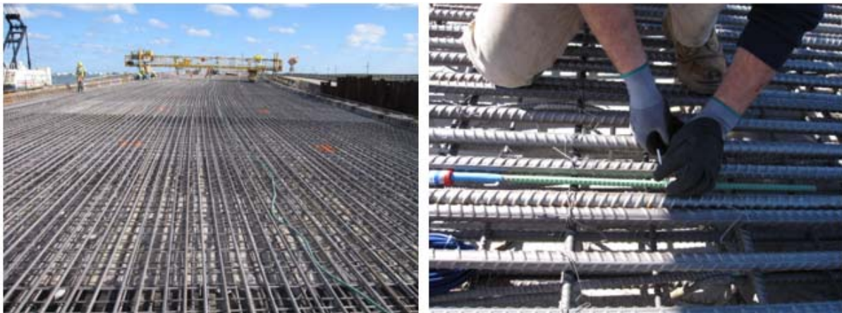
Figure 18 Sensor installation
