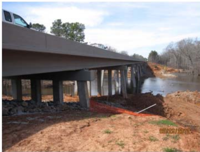
Figure 30 Bodcau Bayou integral abutment bridge
