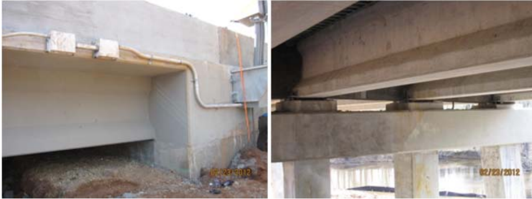
Figure 32 Connections between end abutments and interior bents
