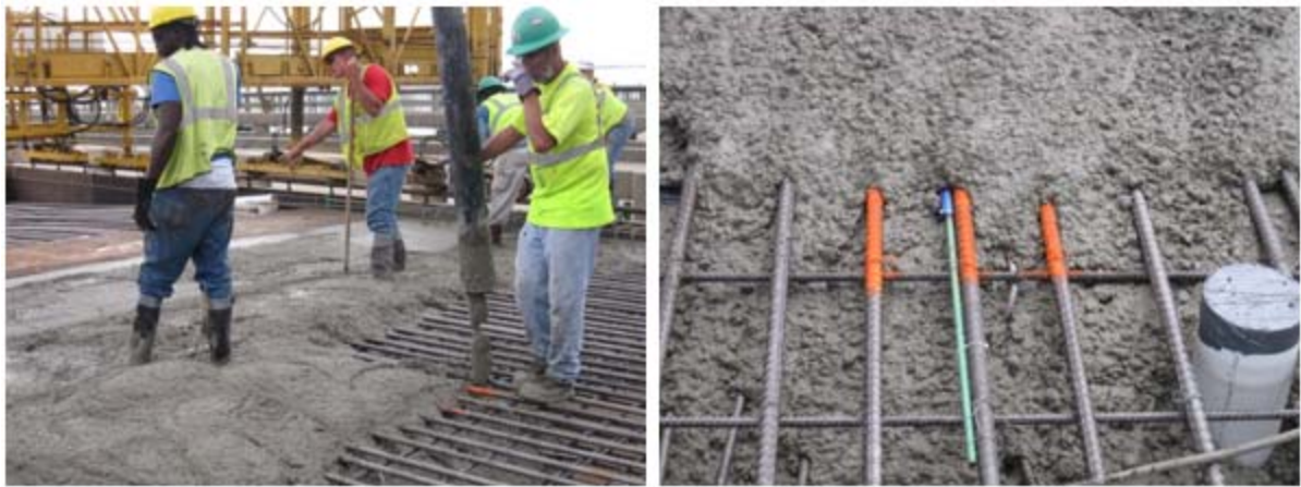
Figure 19 Concrete placement
