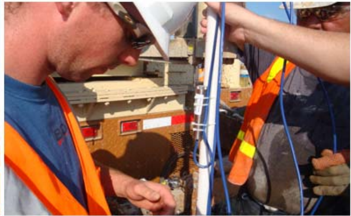
Figure 11 Installation of piezometers
