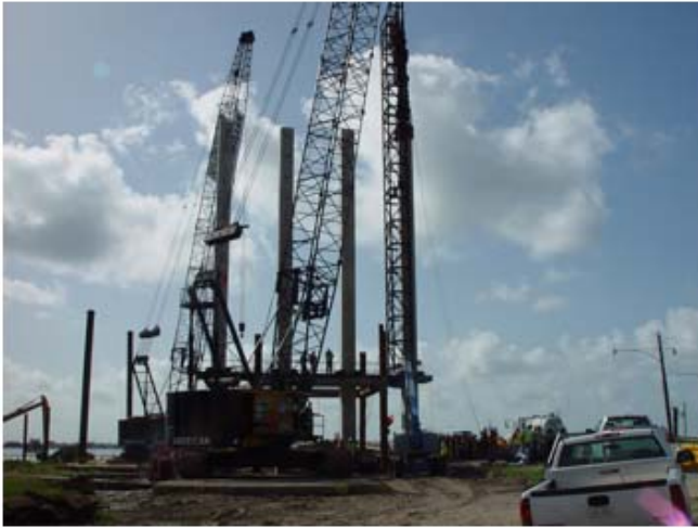
Figure 10 Pile driving at Caminada Bay Bridge
