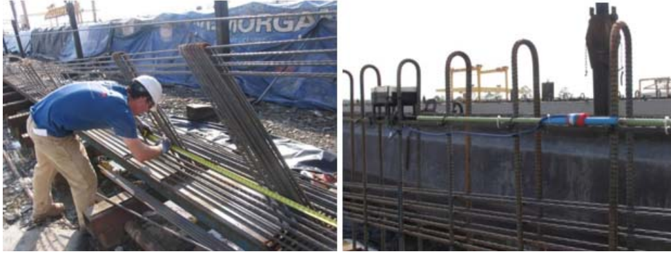
Figure 29 Sisterbar strain gages embedded in the PPC beams
