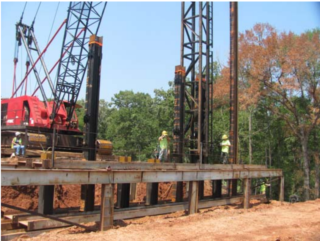
Figure 23 Pile driving at Bodcau Bayou Bridge site
