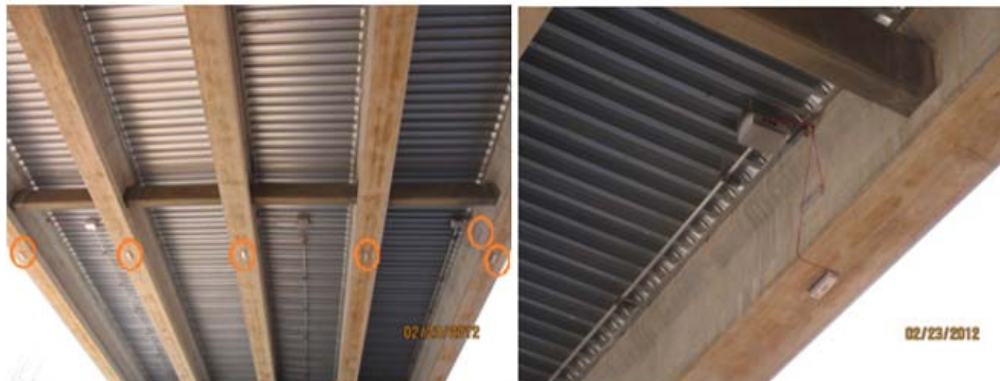
Figure 31 Strain gages applied on the bottom and side surfaces of beams
