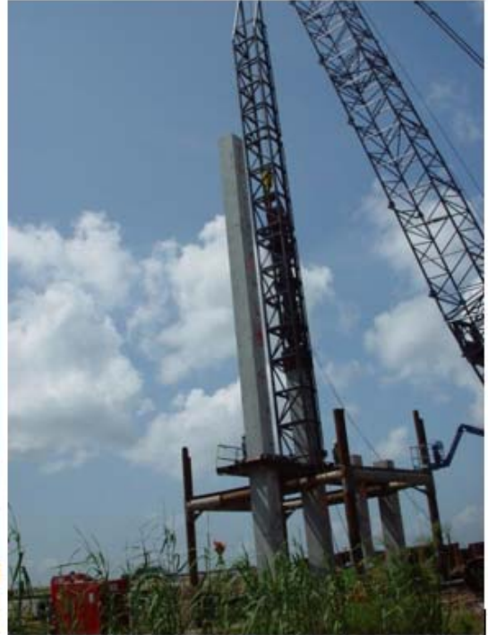
Figure 10 Pile driving at Caminada Bay Bridge
