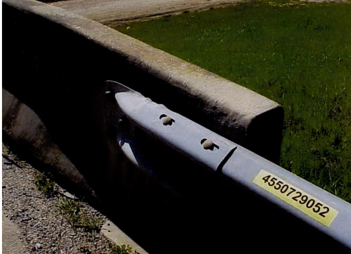
Figure 16B Test site in DeSoto Parish, LA
