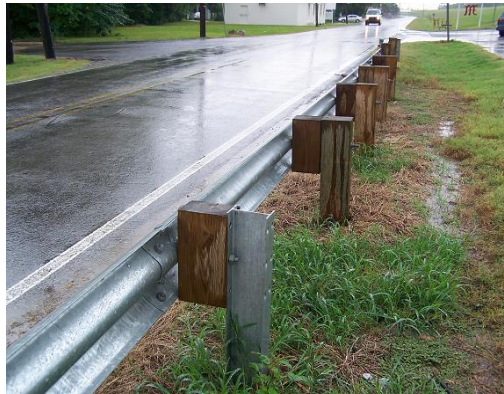
Figure 1 Highway guardrail assembly
