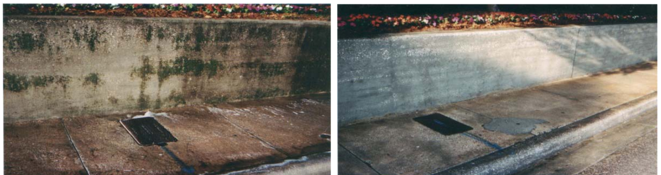
Figure 8 Concrete colonized by algal species (green algae); before and after cleaning [23]
