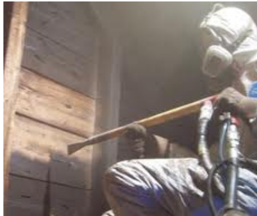
Figure 20 Dry-Ice blasting process [40]
