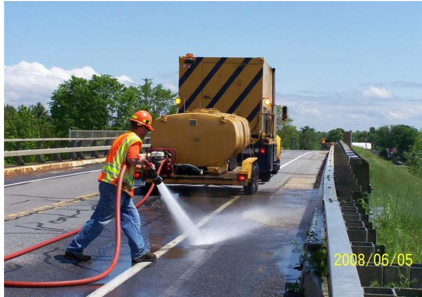
Figure 22 Pressure washing of a concrete deck [41]
