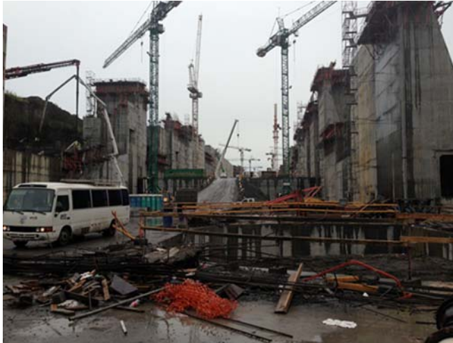
Figure 3 PCE under construction
