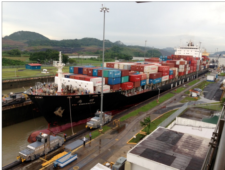
Figure 1 Existing Panama Canal Locks
