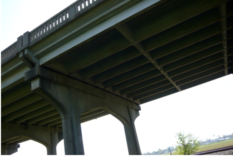
Figure 12 Steel span and concrete span
