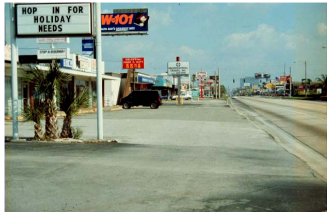
Figure 8: Corridor with no access management policies implemented. Photo source: Williams, K (2003). Access Management. Center for Urban Transportation Research. Retrieved from: http://www.nctr.usf.edu/clearinghouse/netconference/access082003/Kristine%20Williams.pdf
