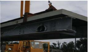
Figure 1 . Old damaged steel grid deck and new FRP-wrapped balsa wood deck
