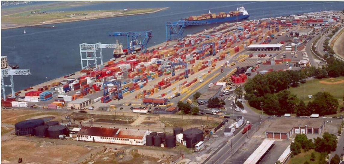
Figure 20 Port of Boston's Conley Terminal (Source: MPA, 2013)
