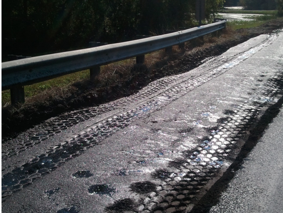
Figure 9 Wet slag-BCS with pumping issue
