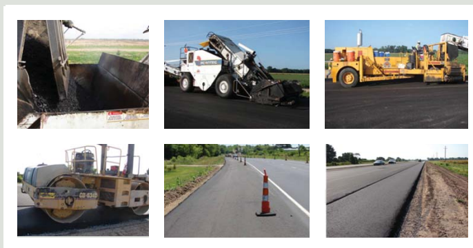
Construction of asphalt treated mixtures layers
