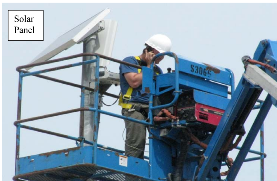
Figure 5 Installation of solar panel and the camera
