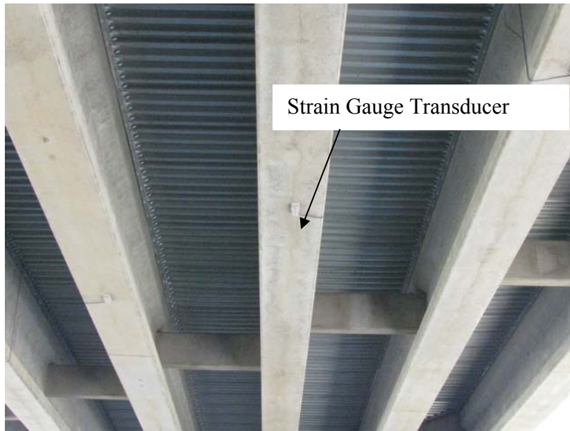
Figure 8 Photo of strain gauge installed in the field
