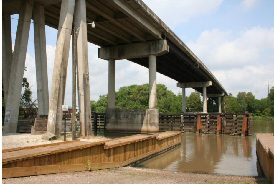
Figure 6 Mermentau River Bridge on US 90 (built in 1980)
