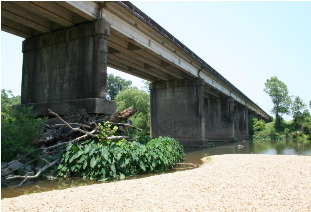
Figure 2 Bogue Chitto River Bridge (built in 1967)
