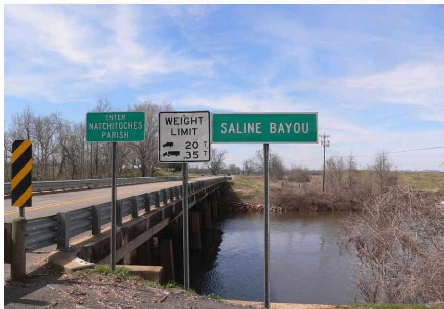
Figure 8 Saline Bayou Bridge (built in 1956)
