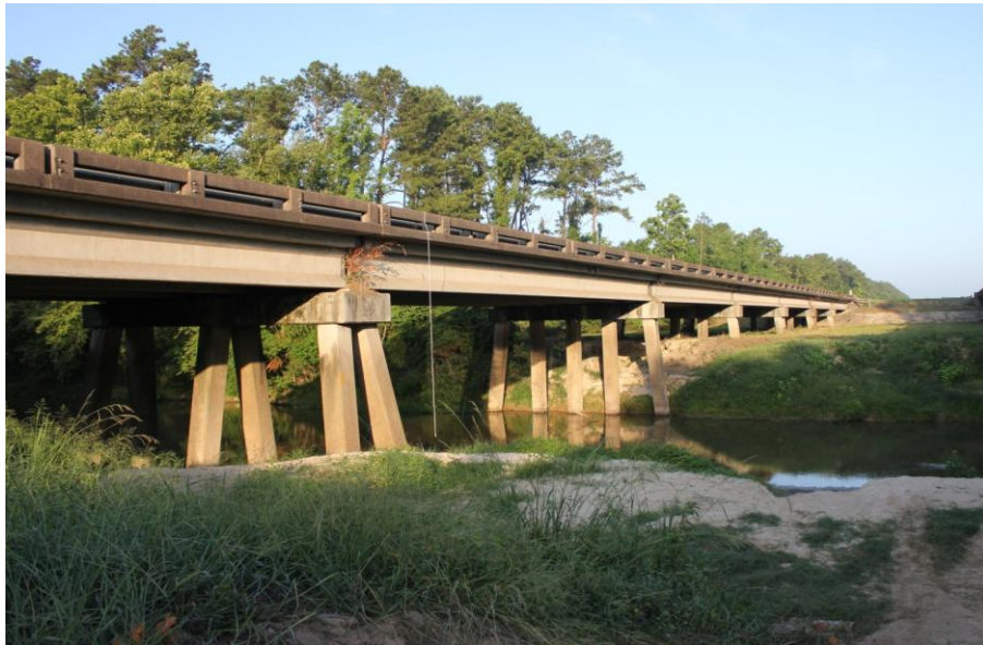
Figure 4 Tickfaw River Bridge on I-12 (built in 1969)
