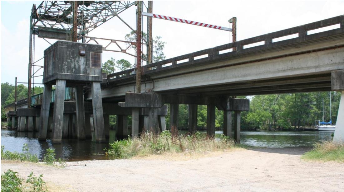
Figure 10 West Fork Calcasieu River Bridge (built in 1968)
