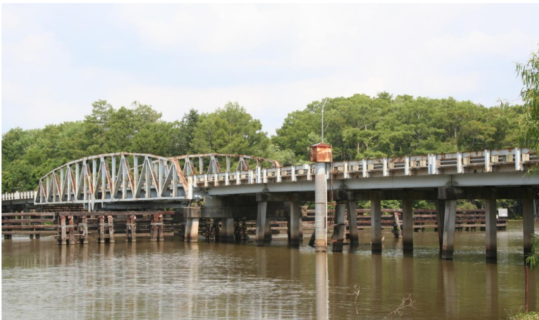
Figure 12 Bayou Lacassine Bridge (built in 1959)
