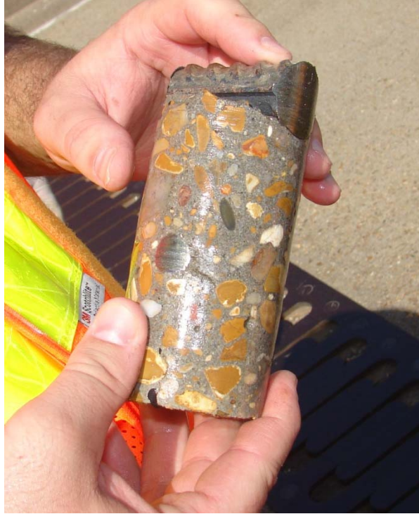
Figure 5 Full depth core showing no steel corrosion
