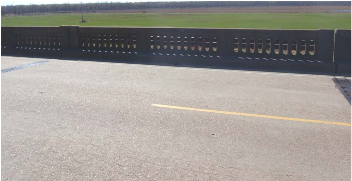
Figure 1 Span 99 looking west (Northbound lane is closest)
