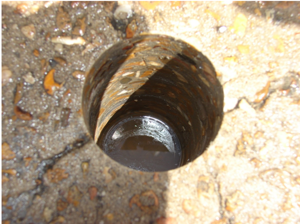
Figure 3 Cracked deck in span 99 northbound (Note the crack depth here was about 2.5 inches)
