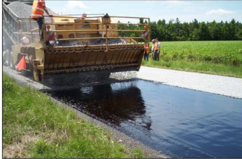
Figure 7 Application of a stress absorbing membrane interlayer [41]
