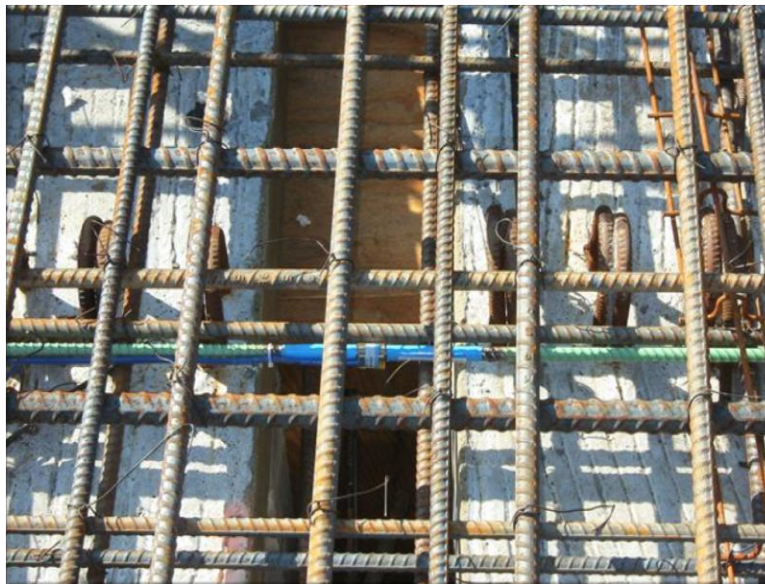
Figure 46 Sisterbars installed next to reinforcing bars in deck over continuity diaphragm
