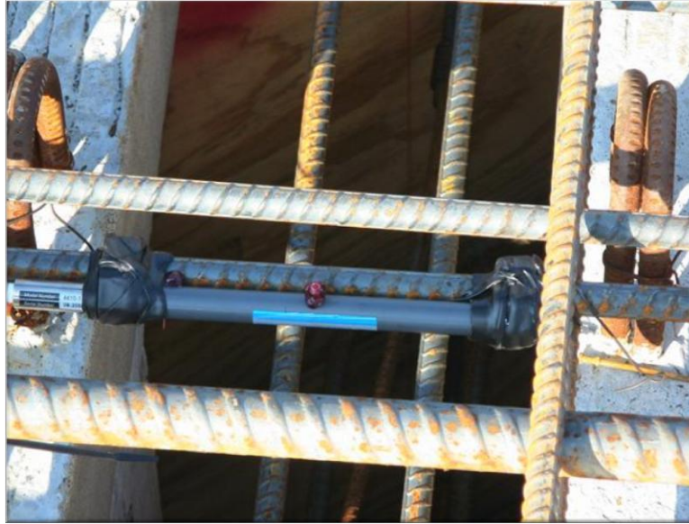
Figure 45 Strandmeters installed on reinforcing bars in deck over continuity diaphragm
