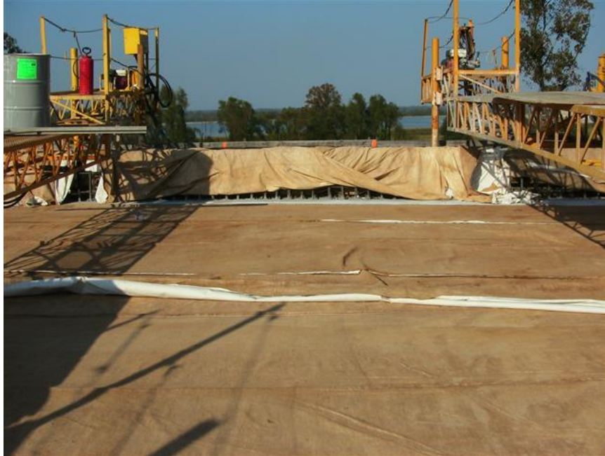
Figure 55 Curing of bridge deck
