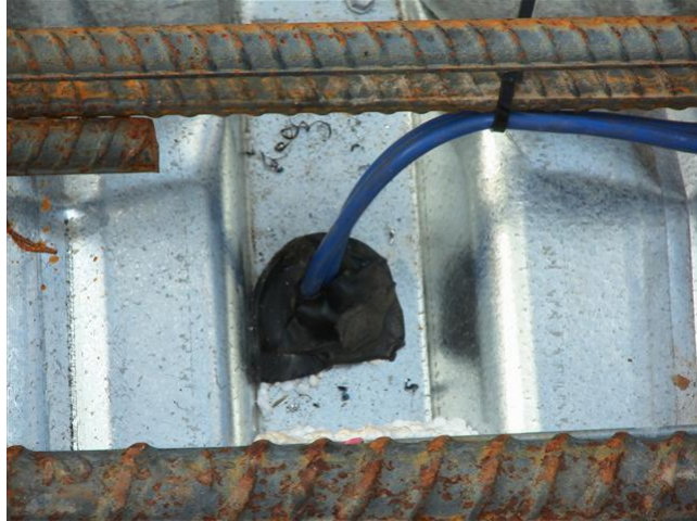
Figure 49 Protection of wiring for embedded sensors prior to concrete casting
