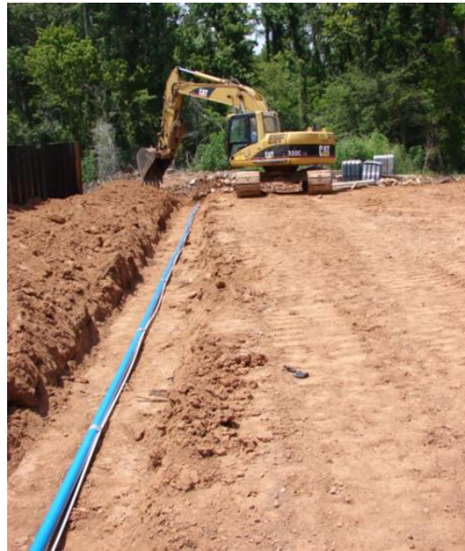
Figure 16 Installation of horizontal inclinometer casing and return pipe
