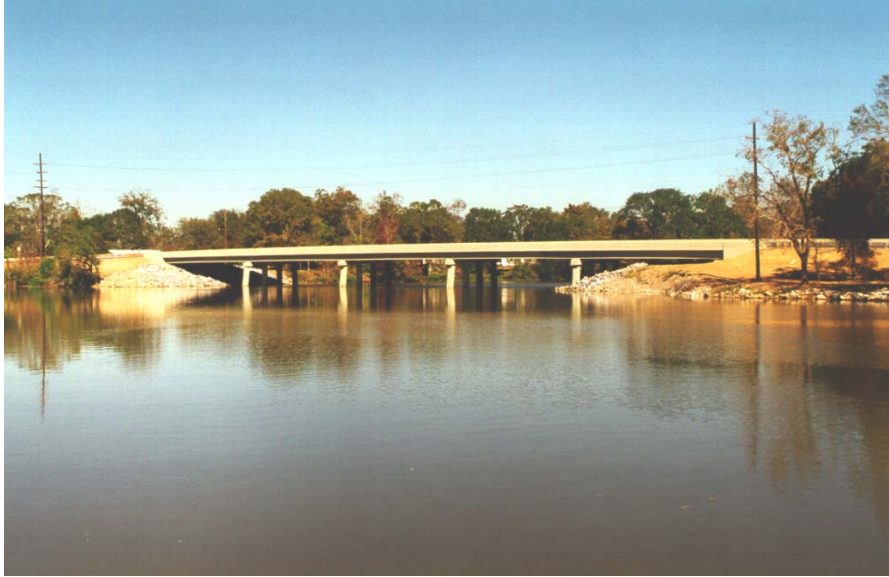
Figure 2 New Charenton Canal Bridge
