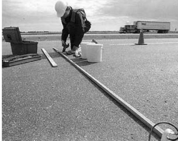
Figure 3 Piezoelectric scale layout [12]
