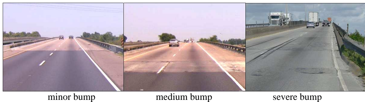
Figure 12 Bridge approach slabs
